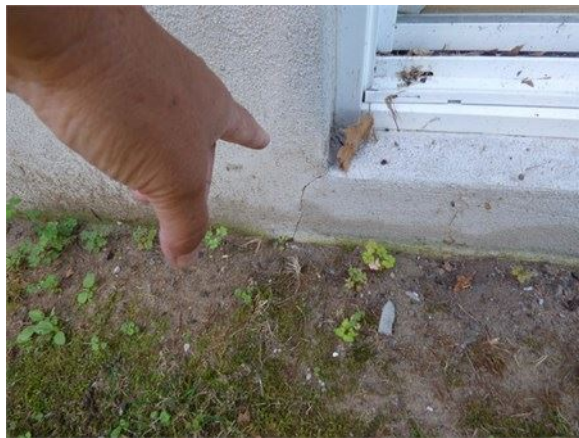
Concrete - Minor fissures to be repaired ( less than1 mm )
