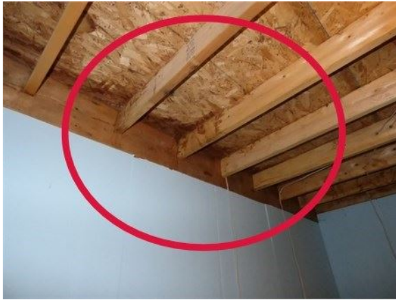
Cold room - Signs of previous water damage noted. Dry at time of inspection. We recommend repairs be performed.
