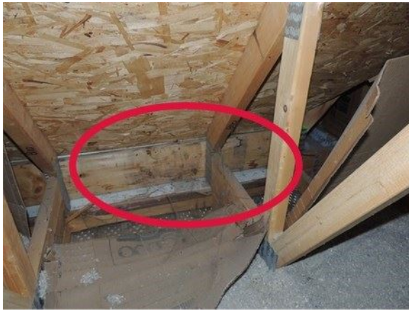
Cold room - Signs of previous water damage noted. Dry at time of inspection. We recommend repairs be performed.
