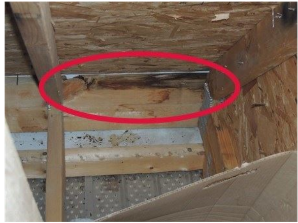
Cold room - Signs of previous water damage noted. Dry at time of inspection. We recommend repairs be performed.
