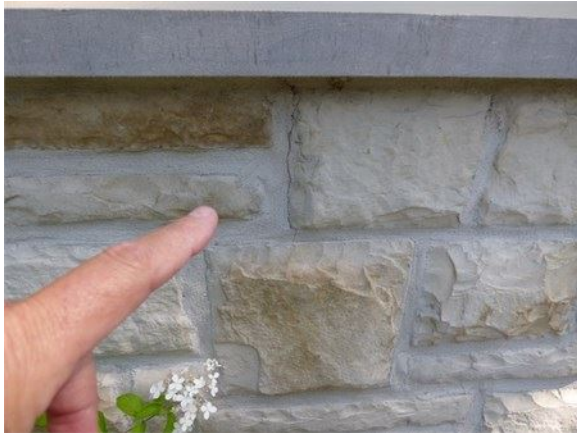
Monitor small cracks.
