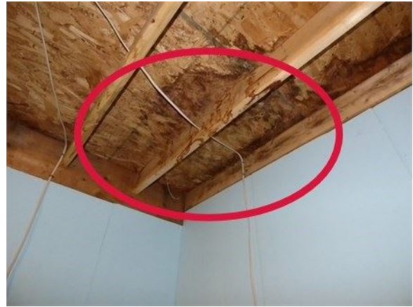
Cold room - Signs of previous water damage noted. Dry at time of inspection. We recommend repairs be performed.
